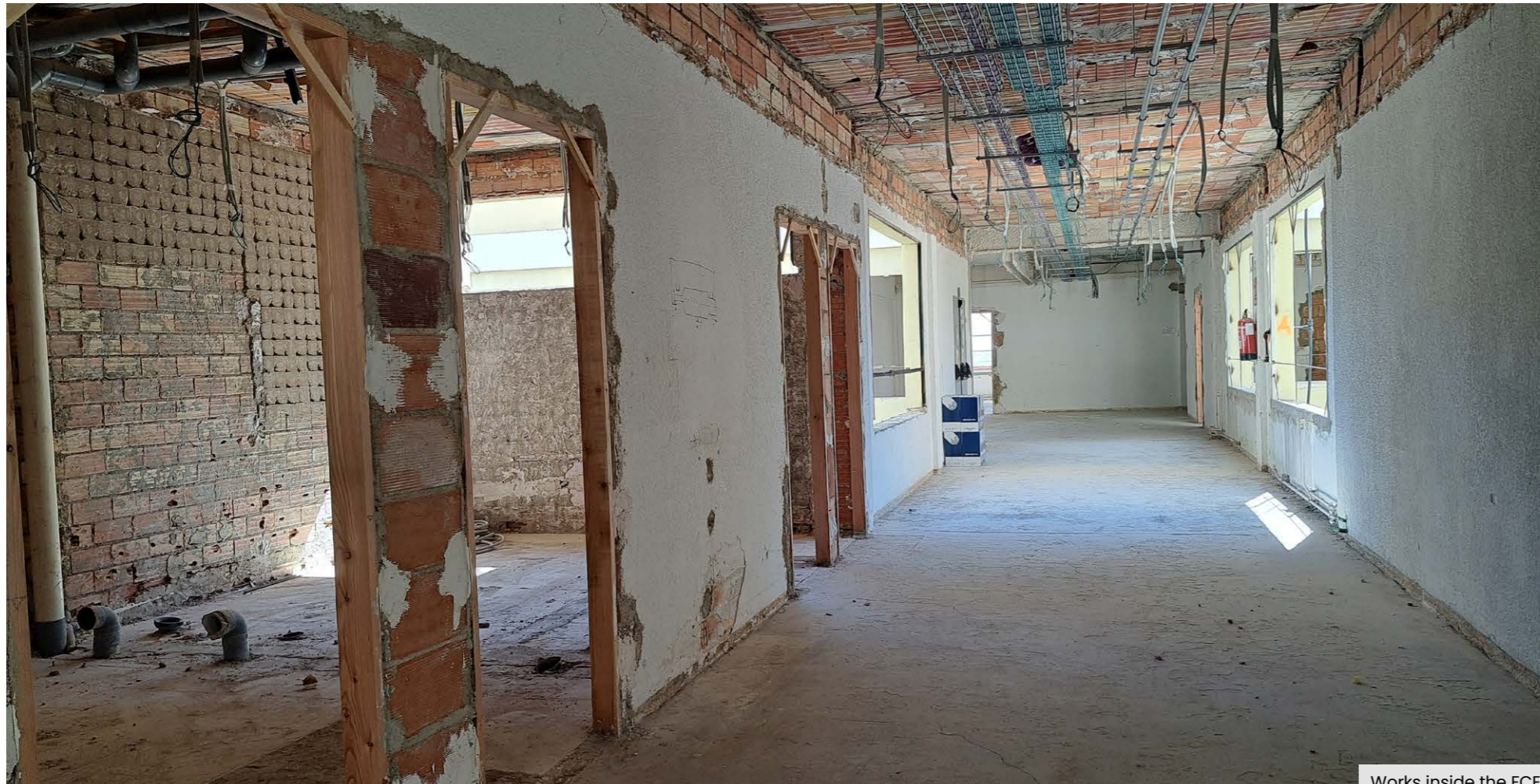
Works inside the FCEP.
